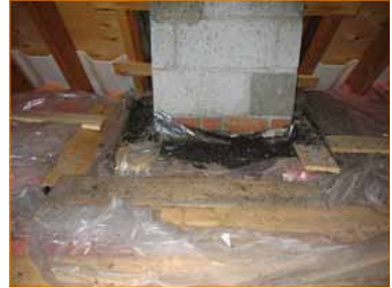
MODIFICATIONS FOR BAT ROOST SITES: PLASTIC SHEETING IN ATTIC TO FACILITATE GUANO REMOVAL AND REDUCE SMELL. PHOTO CREDIT JULIET CRAIG.
